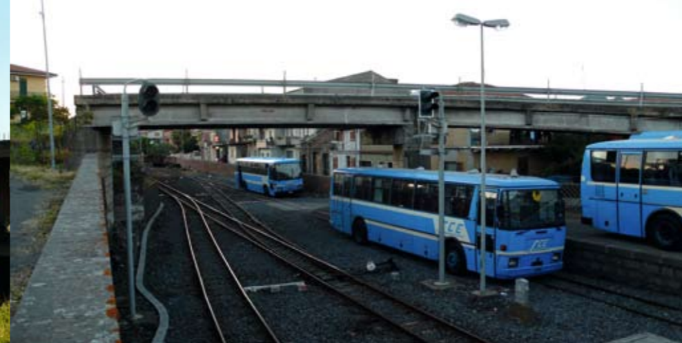
Adrano (Catania). Ponte / Bridge
